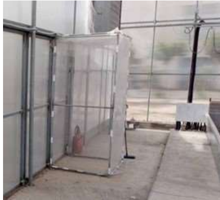
Picture 10. Entrance in the solar drying unit with insect protection
